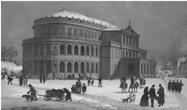
The first Dresden Court opera house, built by Gottfried Semper in 1841
